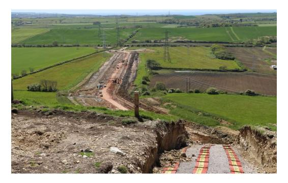
National Grid also carried out the Hinkley Point C Connection Project through the Mendip Hills which again was 400KV cables and again their literature confirms that a working area of only 65m <sup>(30)</sup> was required. The following image shows the actual cables connecting into a jointing box on one of the lines (note that the circuit cables are laid in line here rather than the more compact trefoil arrangement as proposed for the Scheme).
